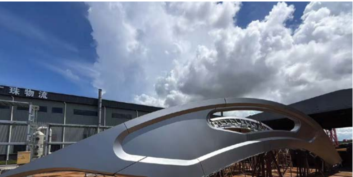
皇冠區域：雙曲面倒角造型鋼架的精準成型 Crown Balcony: Precision fabrication of double-curved chamfered steel framework
