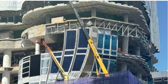
裙底區域：雙曲面單元化幕牆的高空吊裝 Belly Zone: High-altitude installation of the double-curved unitized curtain wall
