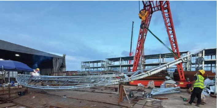
皇冠區域：雙曲面造型鋁板的廠房預裝與精密檢驗 Crown Balcony: Factory pre-assembly and precision verification of the double-curved feature cladding
